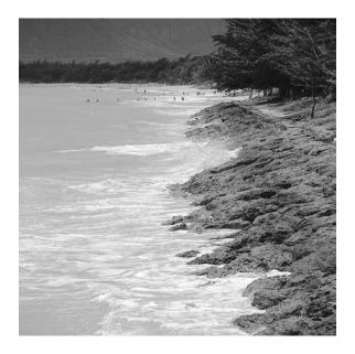
**Waimanalo, Oahu.** Sand impoundment behind this revetment at Bellows Airfield creates a local sand deficiency. As a result, it is responsible for  $\sim$ 1000 ft of beach loss and dune destruction, and chronic erosion characterizes the coast to either side of this structure.
