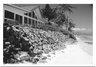
Windward Oahu. Coastal development, besieged by chronic erosion, has historically relied on shoreline hardening for protection. In many cases this has caused beach narrowing, beach and dune loss, and has restricted public access along miles of the Hawaiian coast. COEMAP provides a framework for decisionmaking and implementation to better manage the problem of coastal erosion and to improve the conservation of our beaches and dunes.
