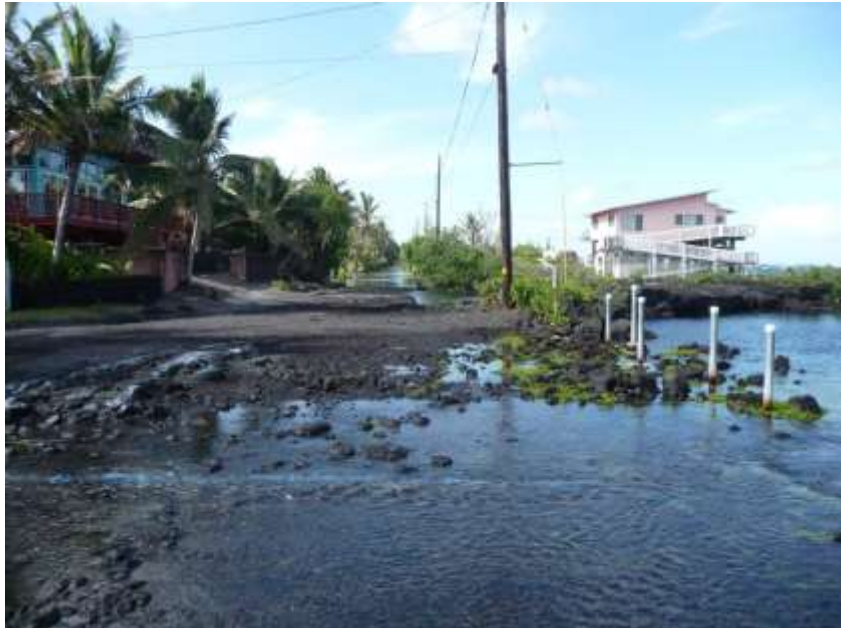
Figure 1 Inland flooding in Puna at high tide.
