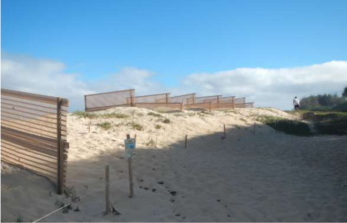
Above: Wind fences installed to gather and maintain sand on dunes. Below: A restored dune with native vegetation.
