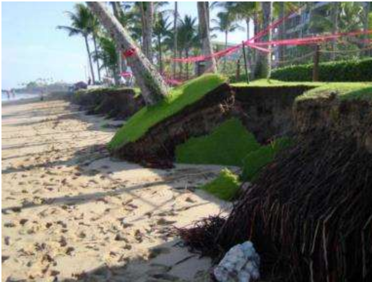
An example of dune grading and subsequent coastal erosion.
