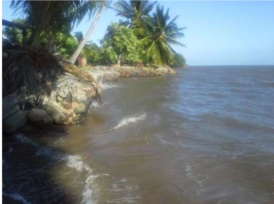
Figure 3 Shoreline armoring along the south shore of Moloka'i.
